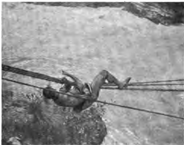
NATIVE CROSSING ROPE BRIDGE
