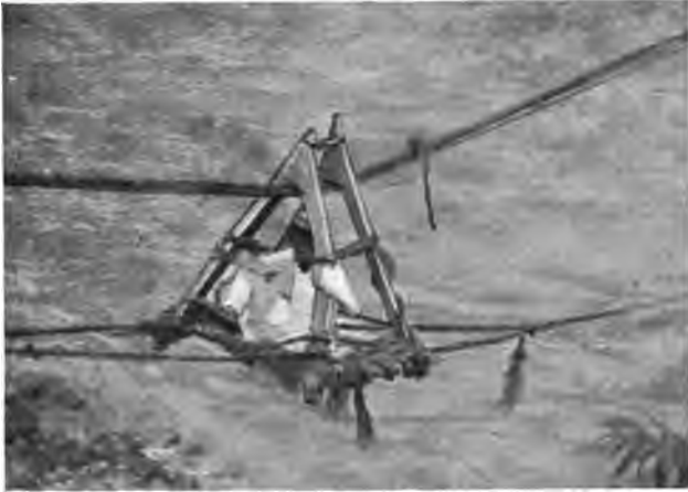
CRADLE ON ROPE BRIDGE
